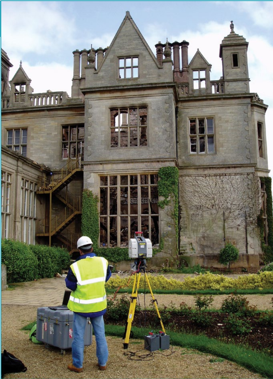
Figure 3 Stoke Rochford Project—Historic Manor damaged by fire, not safe for traditional survey, scanned to assess damage and recovery options (Image courtesy of Plowman Craven)
