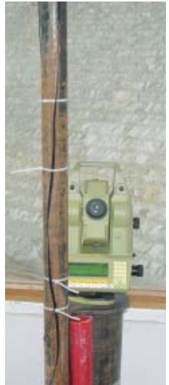
From the safety of the shelter, a Leica TCA 1800 automatically surveys hundreds of retroreflector targets installed on the walls and pit benches.
